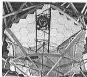
The Hobby-Eberly telescope mirror has 91 segments.
